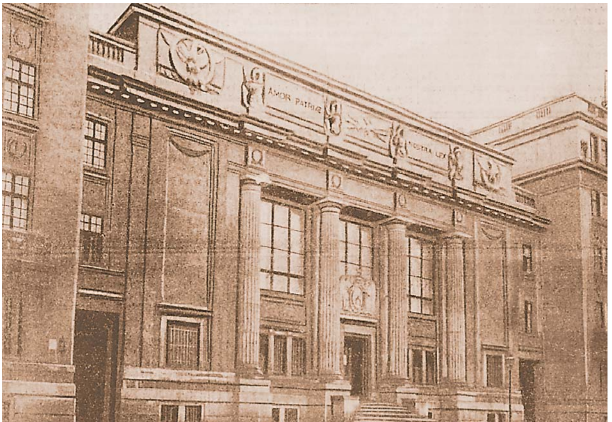
The Krasieński Estate Library in Warsaw (Okólnik Street), before 1930
