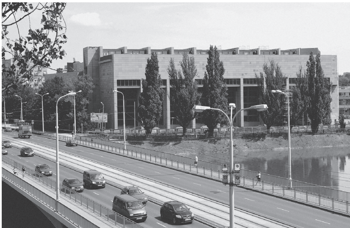
The Wrocław University Library new headquarters
